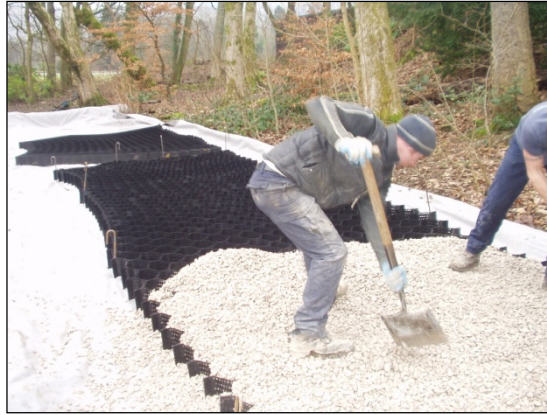
Photo 3- expanding and filling the Cellweb system
