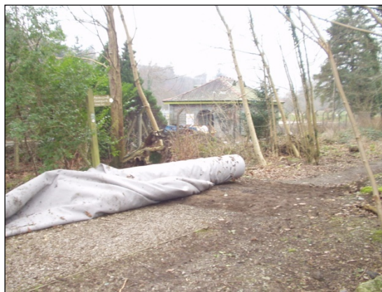
Photo 2- laying of Fibretex material onto existing subgrade
