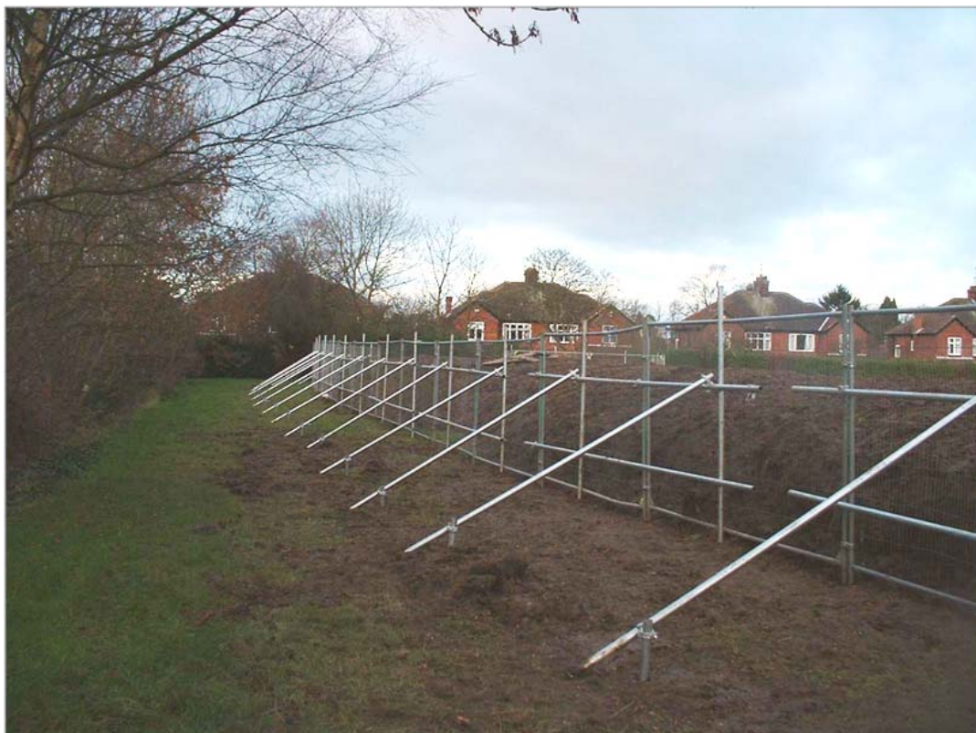
Figure 4 – Actual barrier erected on site
